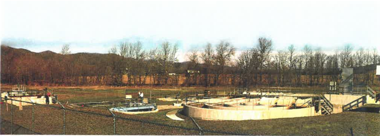
Silling Associates Huttonsville Correctional Center Wastewater Treatment Plant 405 Capitol Street
